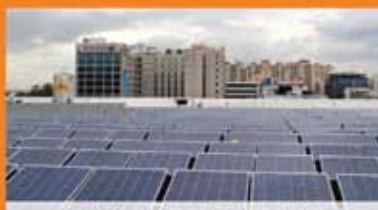
Rooftop Project, Karnataka
