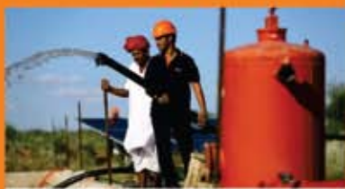
Solar Water Pump Project, Rajasthan
