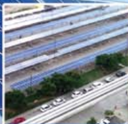
500 kW Carport project at Medanta Medicity, Gurgaon, Haryana
